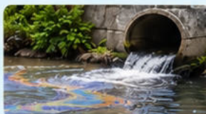
Spills, Leaks & Runoff
